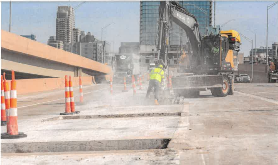
US-131 Concrete Patches; Photo courtesy of MDOT
